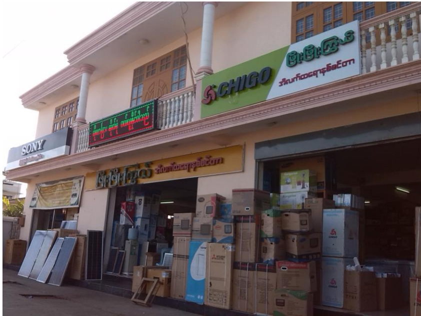
Figure 4. A typical commercial building in Nay Pyi Taw, with long but small column girth at the ground floor (strong beam and weak column building category)
