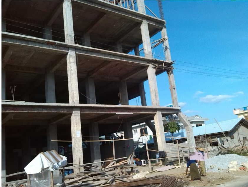
Figure 3. Non-symmetric building with long column at ground floor in Central Business District of Nay Pyi Taw
