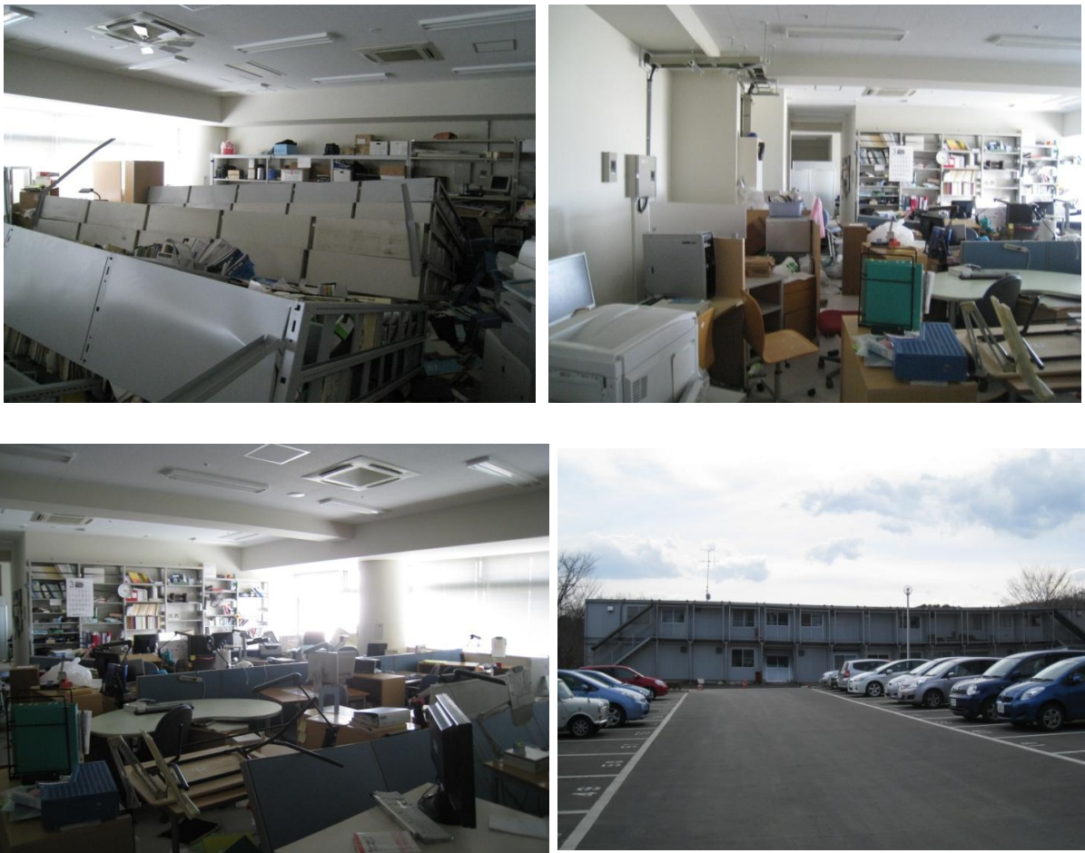
Fig.2 Damage from earthquake
